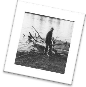
Shoreline during the construction of Green Lakes State Park. Photo by Arvin H. Almquist. Digitized by Fayetteville Free Library (Almquist Green Lakes Collection)
